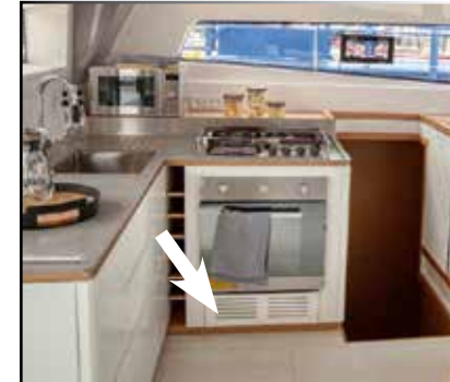
LOCATION OF THE GAS VALVES
