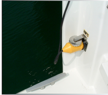
SHORE POWER SOCKET
