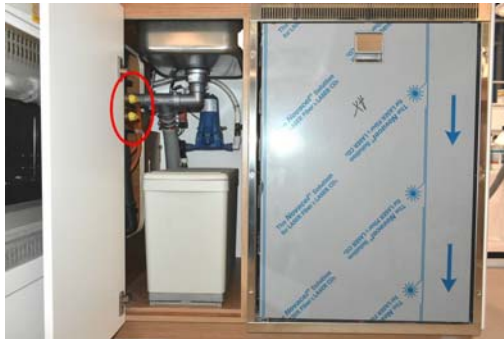
Gas supply valve Location: beneath the oven
