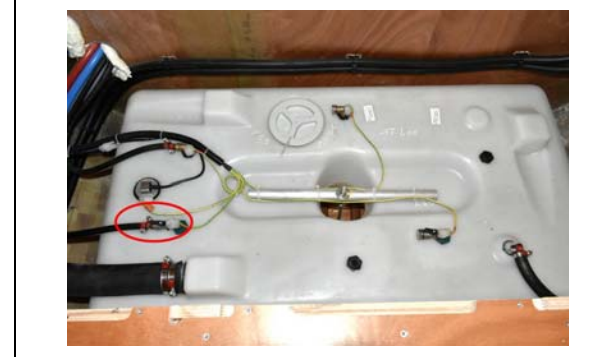
Fuel supply valve located directly on the tank
