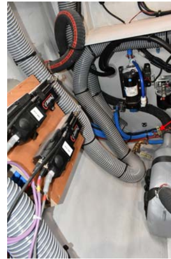
Water tank / water unit supply valve
