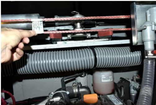
Label indicating the date on which the steering cable should be changed
