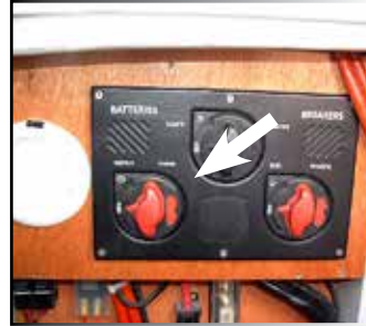
STARBOARD ENGINE CUT OUT
