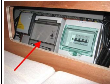
Differential circuit breaker (Ref 3)
