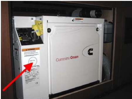
Extinguisher access hole
