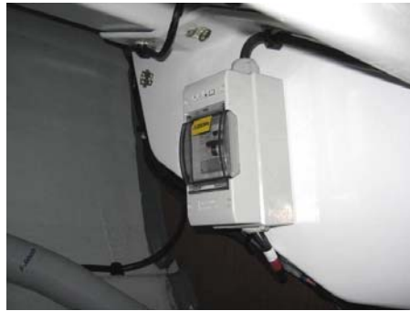
Bipolar circuit breaker (Ref 2)
