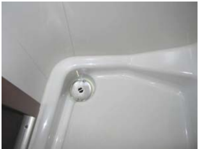
Drainage plug hole - Shower
