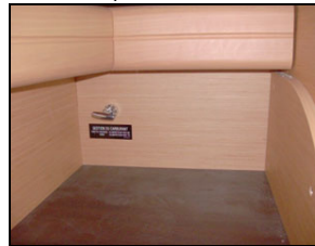
Lever pushed: Port tank
