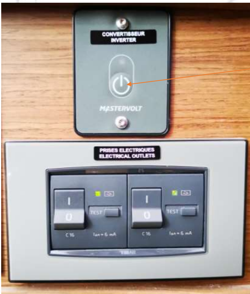
Inverter control & Power button
