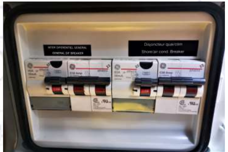
Generator/Shore Power Breakers Behind Generator
