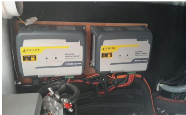
40A battery charger | CRISTEC Charges service batteries and engine
