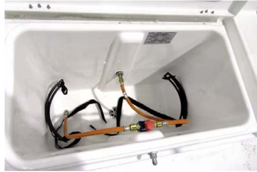
Gas supply valve Location: beneath the oven
