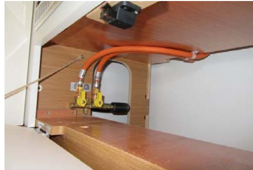
Gas supply valve Location: beneath the oven
